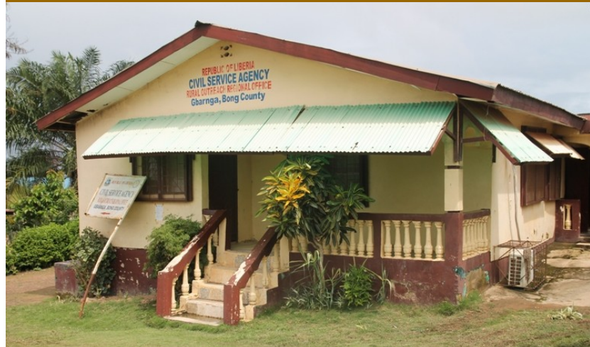
CSA Regional Office (Gbarnga, Bong County)
